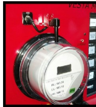
Testing with the Centron Pick-up
